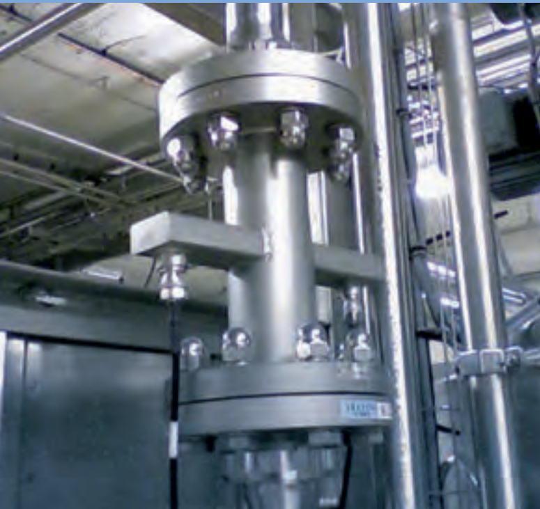
Determining the dry substance in a wastewater pipe – LB 566 with flow cell.
